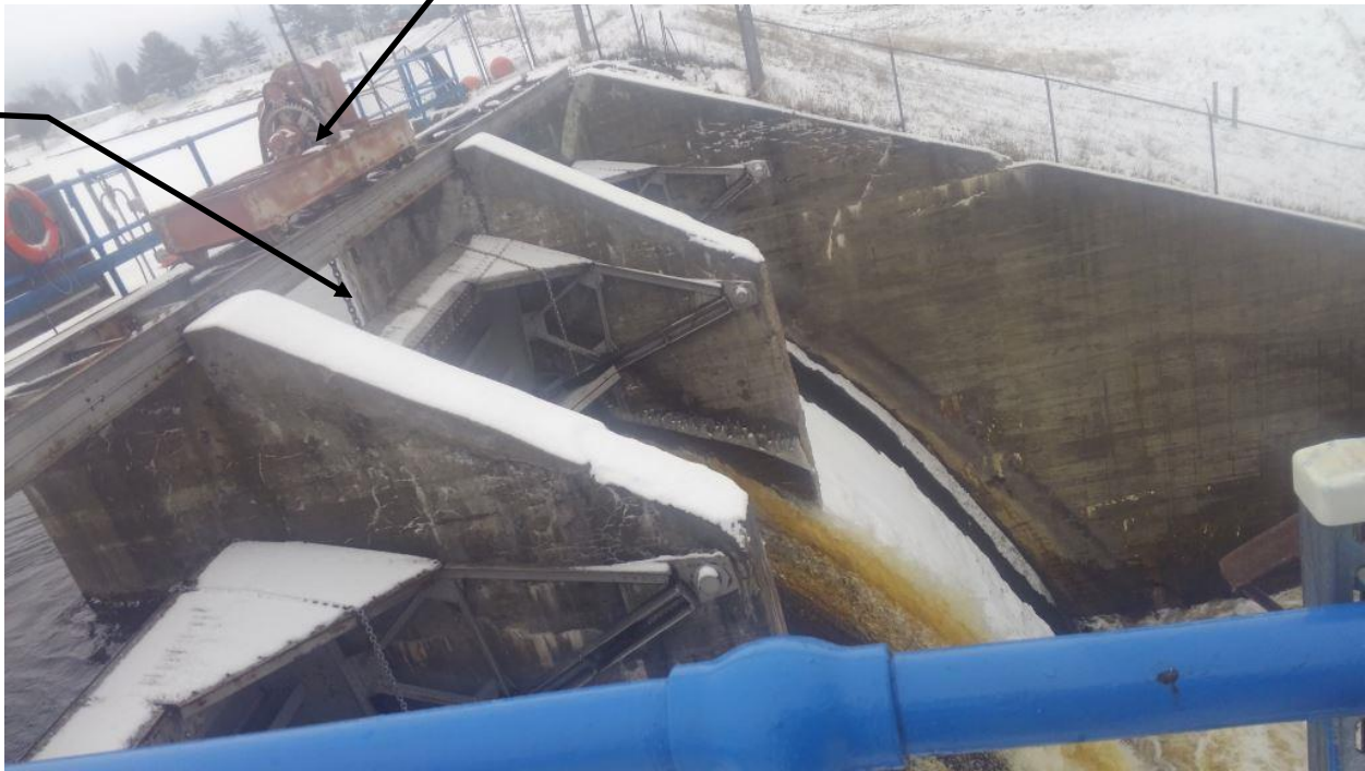
View of Edenville Dam Powerhouse Spillway Gates (22 December, 2017)
